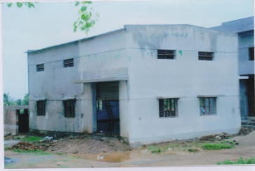
Value addition plant- Building
