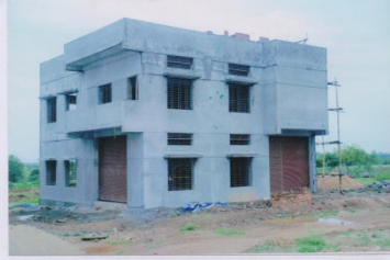
Packing and Testing Reserve Building
